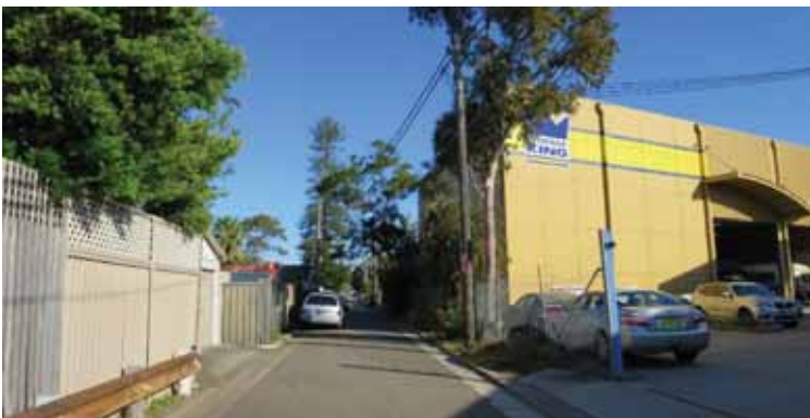
Figure 8: View of Storage King from Roberts Lane
