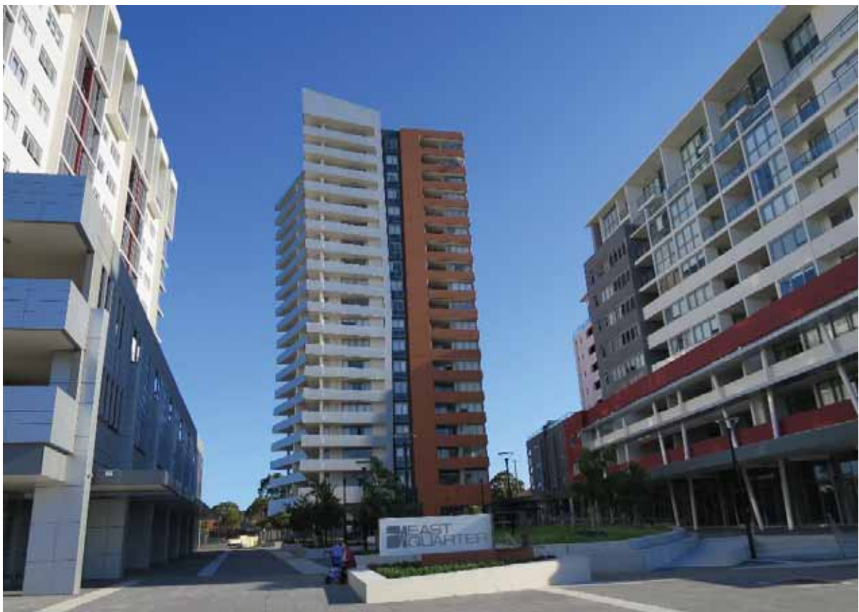
Figure 16: East Quarter development viewed from near Forest Road
