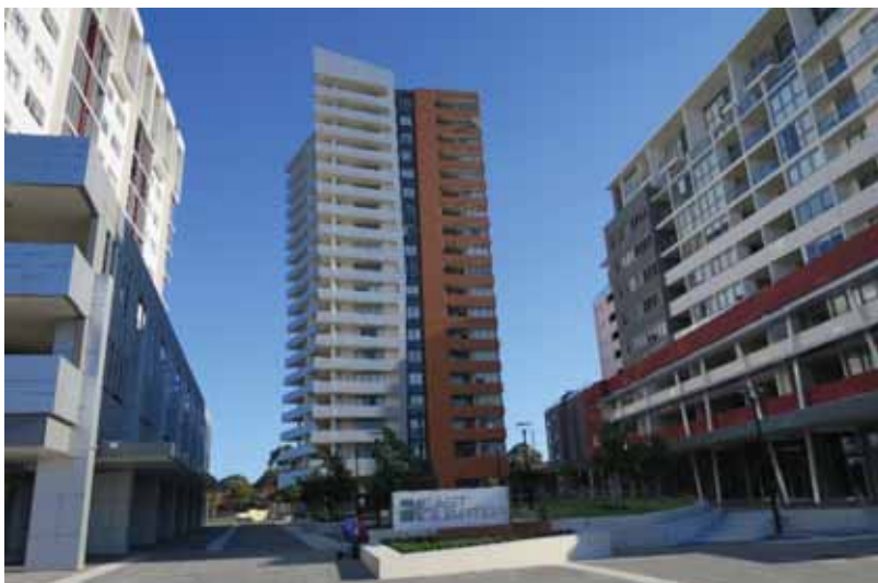
Figure 28: East Quarter development viewed from near Forest Road
